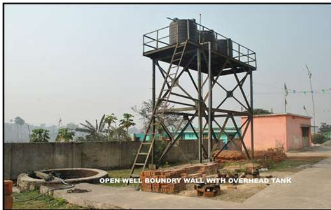
Water supply at Boulpur R&R site
