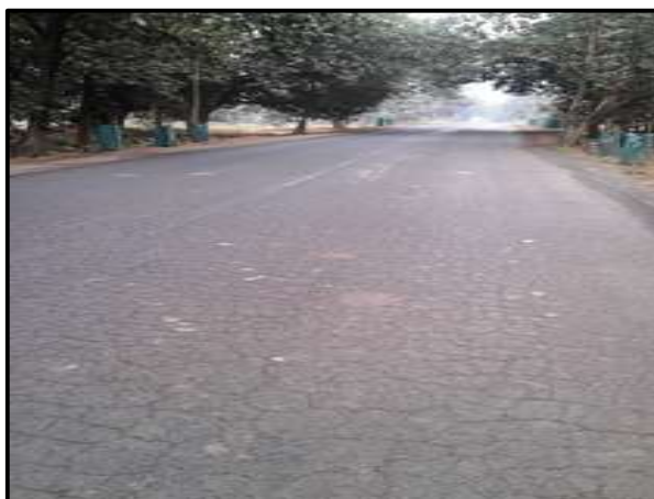
Strengthening of Balinga Tapadia Road (21Km) in Sundergarh district
