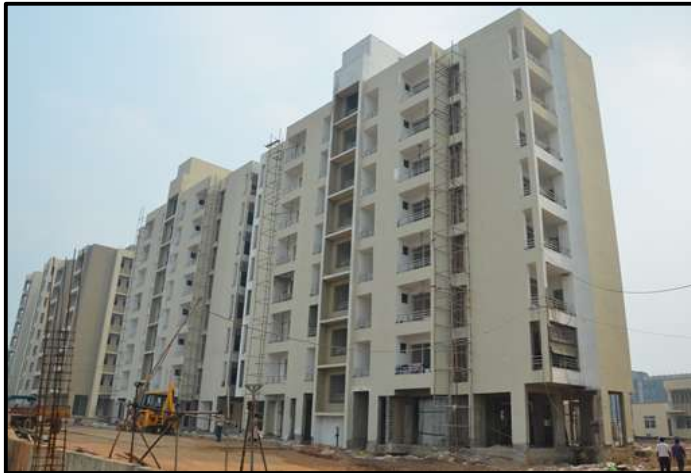
Construction of Medical college at Talcher in progress
